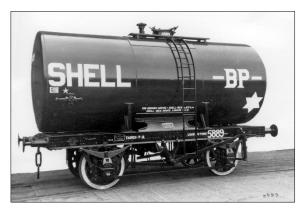
Cylindrical tank wagons similar to examples shown on pages 40, 42-45, 50, 51, 83 (top), 85 (bottom) and 86 (top). This livery seems to have been the most common and was used on a large number of tank wagons of varying designs – just one example is included here (left) (*HMRS photo*).
